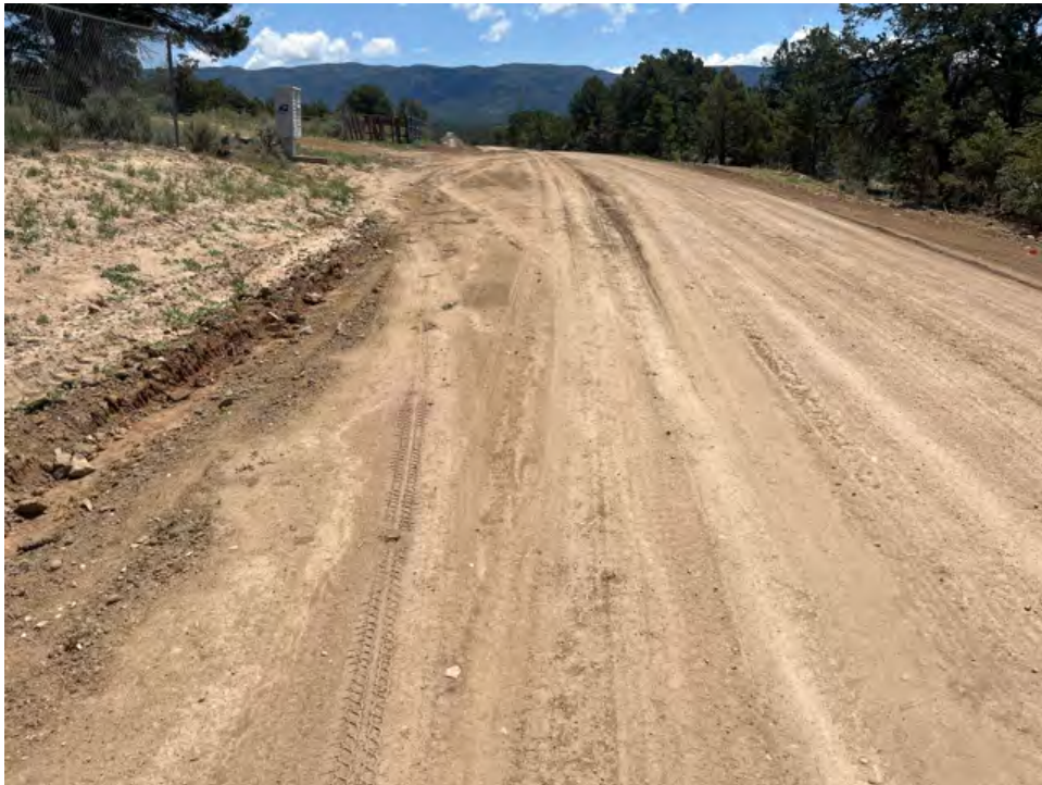
Photo 14-1. Western end of the Naranjo Creek Rd waterline improvement project, looking east.
