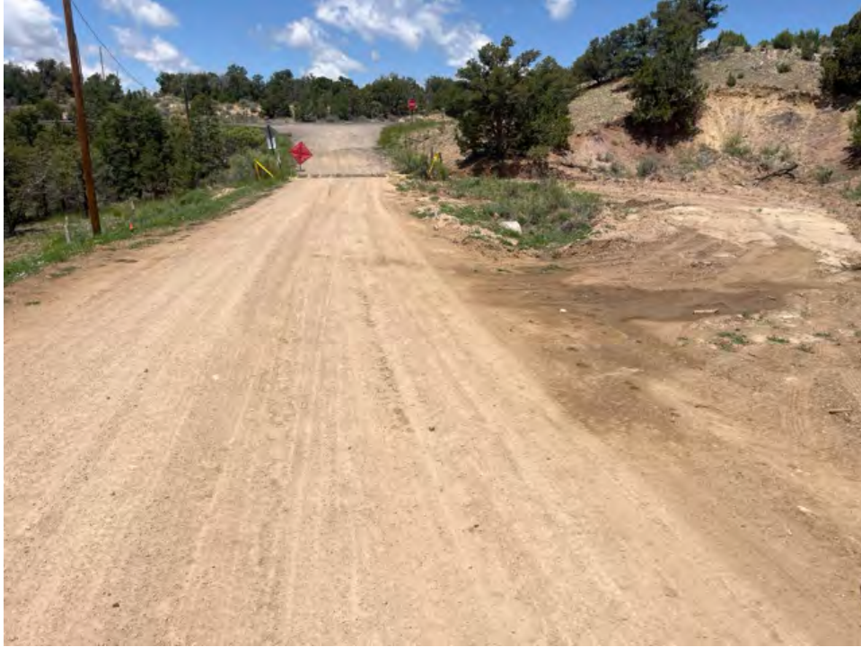
Photo 14-2. Western end of the Naranjo Creek Rd waterline improvement project, looking east.
