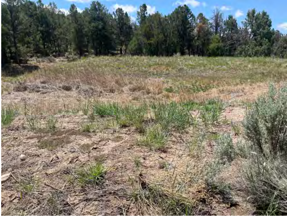
Photo 07-1. Earthen dam water tank along the south side of the Naranjo Creek Rd waterline improvement project.
